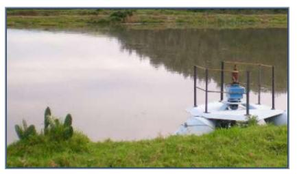
A pond system was constructed for an army base camp in Iraq housing about 1,000 soldiers. The pond system consisted of an inlet works which received the water borne sewage from the camp. This inlet works is equipped with a fine screen unit whereafter the water is discharged to the primary oxidation pond. From the primary pond, the water is treated through a serried of facultative ponds to eventually produce a final effluent which is of sufficient quality to be irrigated onto pastures.
